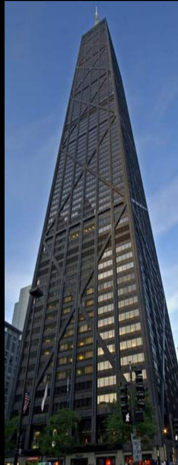
John Hancock Building
