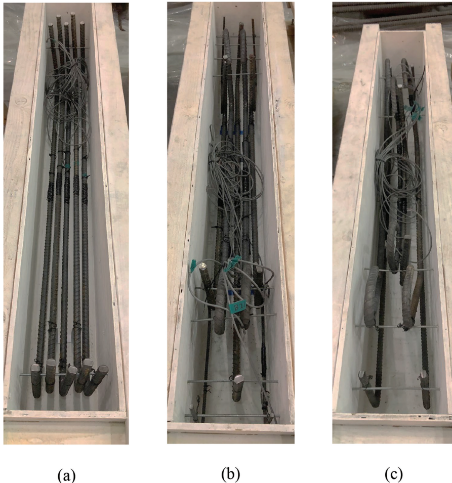
Fig. 8—Steel reinforcement cages used for: (a) ACI layout; (b) optimized layout I; and (c) optimized layout II.
