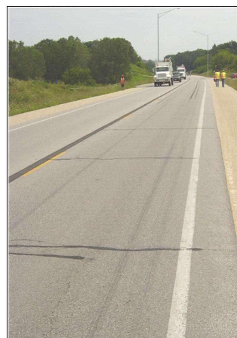
Figure 1: Typical examples of low-temperature cracking
