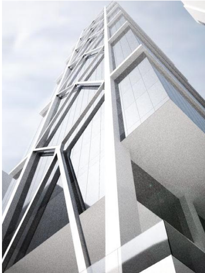
Combining elements for structural braced frames
