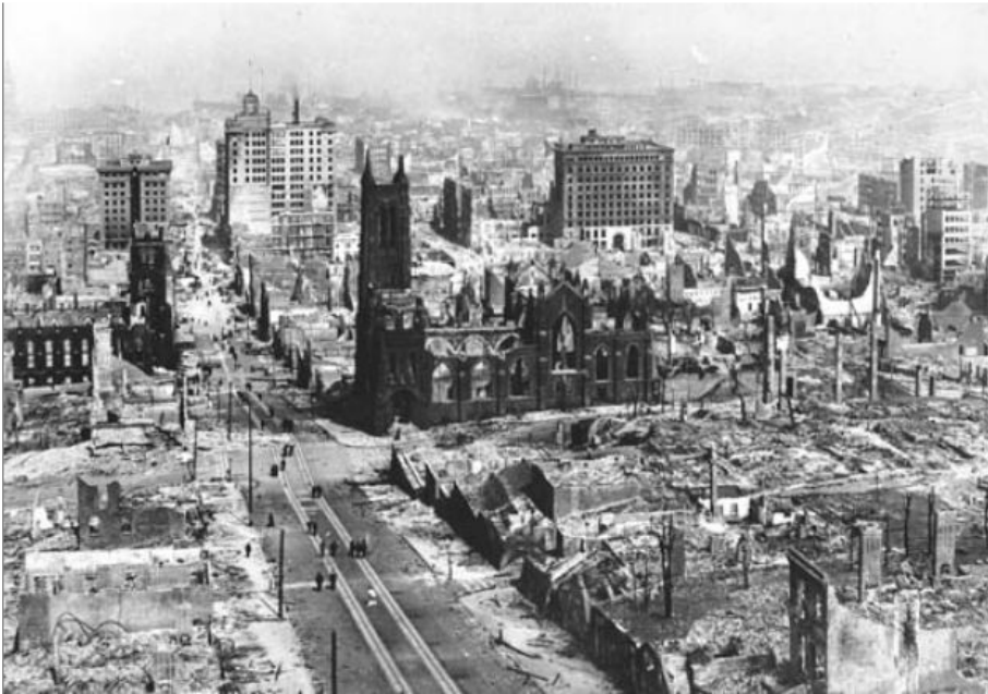
San Francisco Earthquake, 1907
