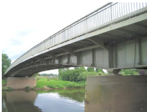
(b) Bridge girder
