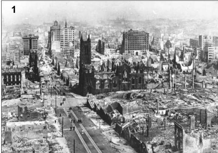
San Francisco Earthquake, 1906
